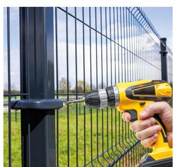
Plastic intermediate clamps should be placed under horizontal bar of fencing panel, and the lower clamp should be placed above horizontal bar. Thus the panel is set stable on clamps. For heights above 1.5m it is recommended to mount 3 sets of clamps.
