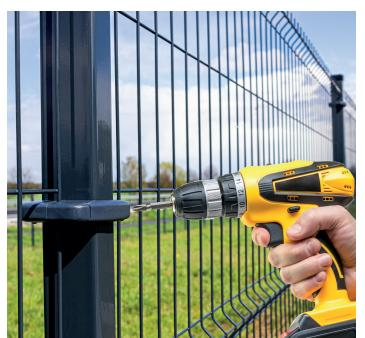
Plastic intermediate clamps should be placed under horizontal bar of fencing panel, and the lower clamp should be placed above horizontal bar. Thus the panel is set stable on clamps. For heights above 1.5m it is recommended to mount 3 sets of clamps.
